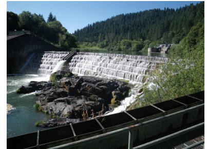
Figure 1. Cape Horn Dam creating Van Arsdale Reservoir. Fish ladder in foreground with water diversion tunnel to Russian River in background.
