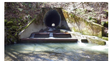
Figure 2. Traditional fish passage structure aimed at assisting salmonid species without consideration of lamprey.
