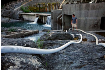
Figure 3. USFWS biologist, Damon Goodman, looks on at recently installed Pacific lamprey passage tubes at Cape
