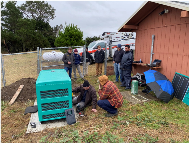
Figure 1. WNRD and contractors finish installation of propane back-up generator at TBR, helping the Reservation be more resilient to power grid failures.
