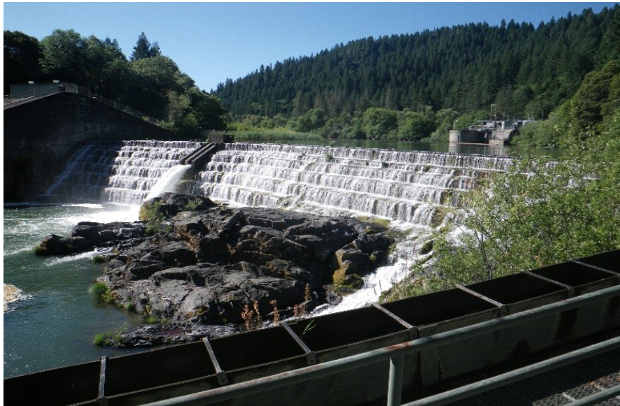
Figure 1. Cape Horn Dam creating Van Arsdale Reservoir. Fish ladder in foreground with water diversion tunnel to Russian River in background.
