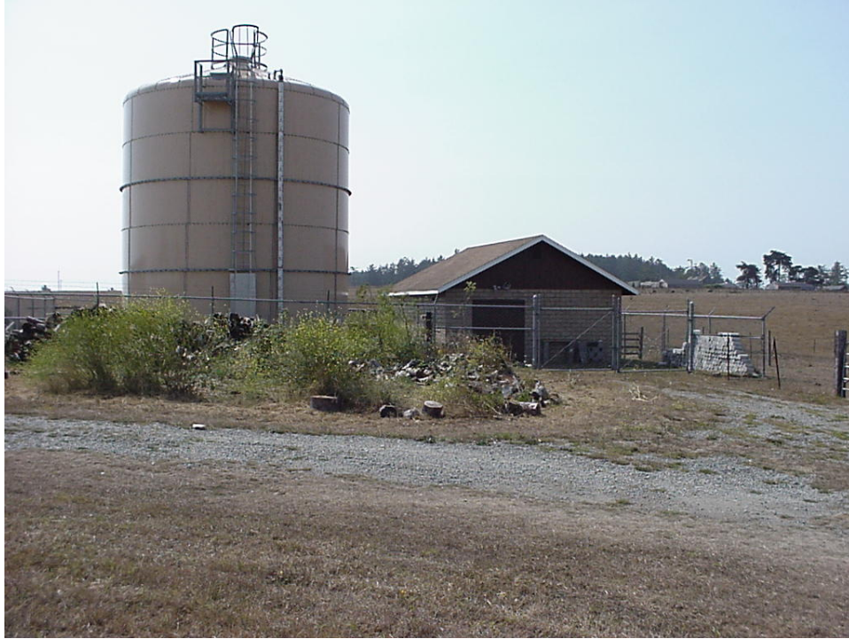
Figure 7. Water Treatment Building. The Table Bluff Reservation community drinking water system includes this treatment building and tank that stores 100,500 gallons of treated groundwater.
