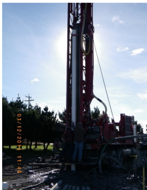
Figures 11 & 12. Drilling Water Wells. In 2008 and 2011, the Tribe installed two drinking water wells on TBR, giving the community access to the higher quality groundwater beneath their feet.
