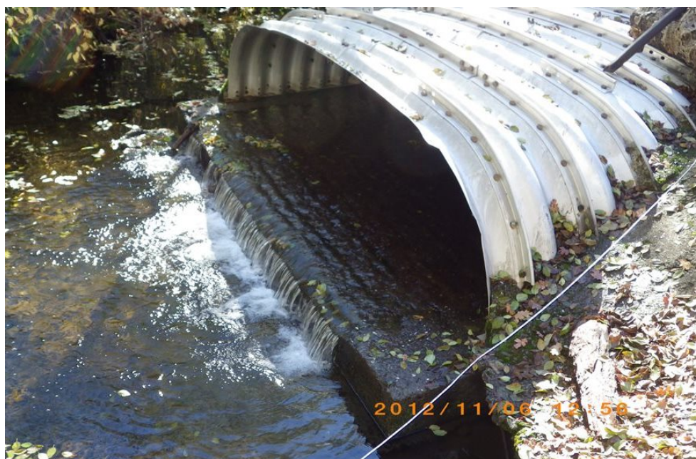
Figure 2-4. Example of culvert outlet apron with a vertical step at a crossing of Butte Creek (PAD 715481).
