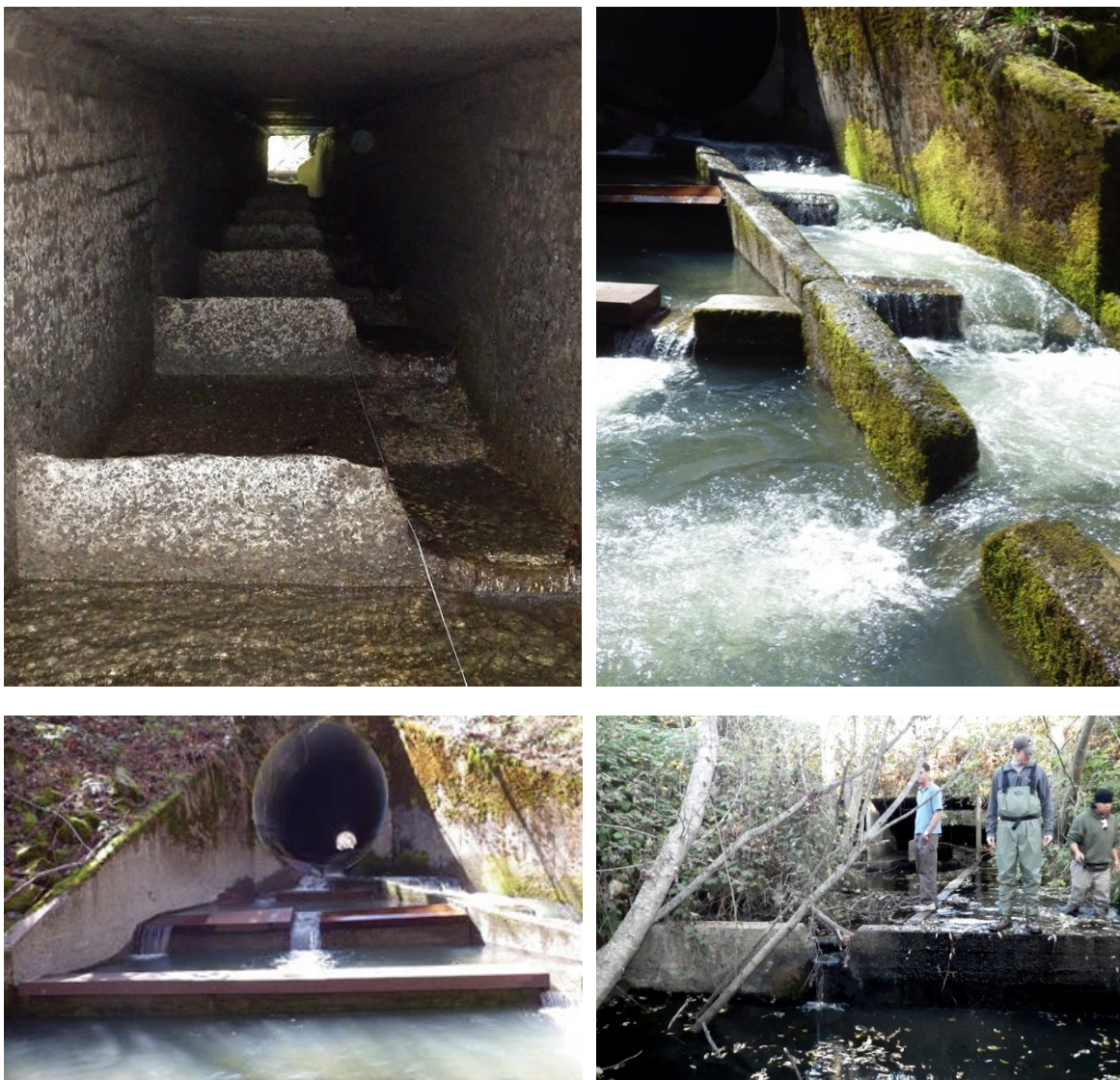
Figure 2-5. Examples of internal structures and modifications at road crossings in the Eel River basin. Internal baffles (top left; Fish Creek, PAD 707157), step-pool fishways at outlet (top right and bottom left; Elk Creek, PAD 707107), and tailwater control weir (bottom right; Rohner Creek at 12 th St. in Fortuna, CA).
