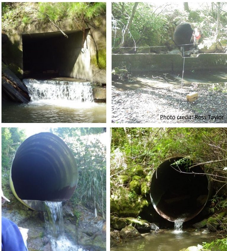
Figure 2-3. Examples of perched road crossings or tailwater control weirs found in the Eel River basin. Clockwise from upper left: Oil Creek (PAD ID 736789), Dinner Creek (PAD ID 723276), Stitz Creek (PAD ID 715449), Strawberry Creek (PAD ID 715429)
