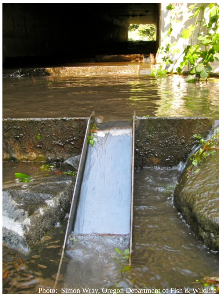
Figure 5-2. Example of installation of lamprey ramps to improve passage in Threemile Creek, Oregon.
