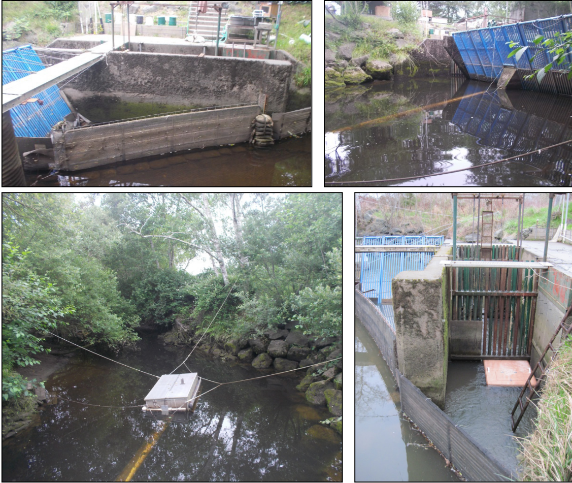
Figure 3. Photos of the HFAC weir and associated traps in lower Freshwater Creek. Top left: looking at upstream edge of weir in foreground and adult salmonid trap in background. Top right: looking at downstream edge of weir and pipe leading to downstream migrant trap. Bottom left: downstream migrant trap below weir. Bottom right: looking downstream at adult salmonid trap with the plywood lamprey box trap in place (Photos by C. Anderson).
